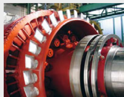
ÖBB'S POWER PLANTS. Rotor of a traction power generator at Braz power plant
