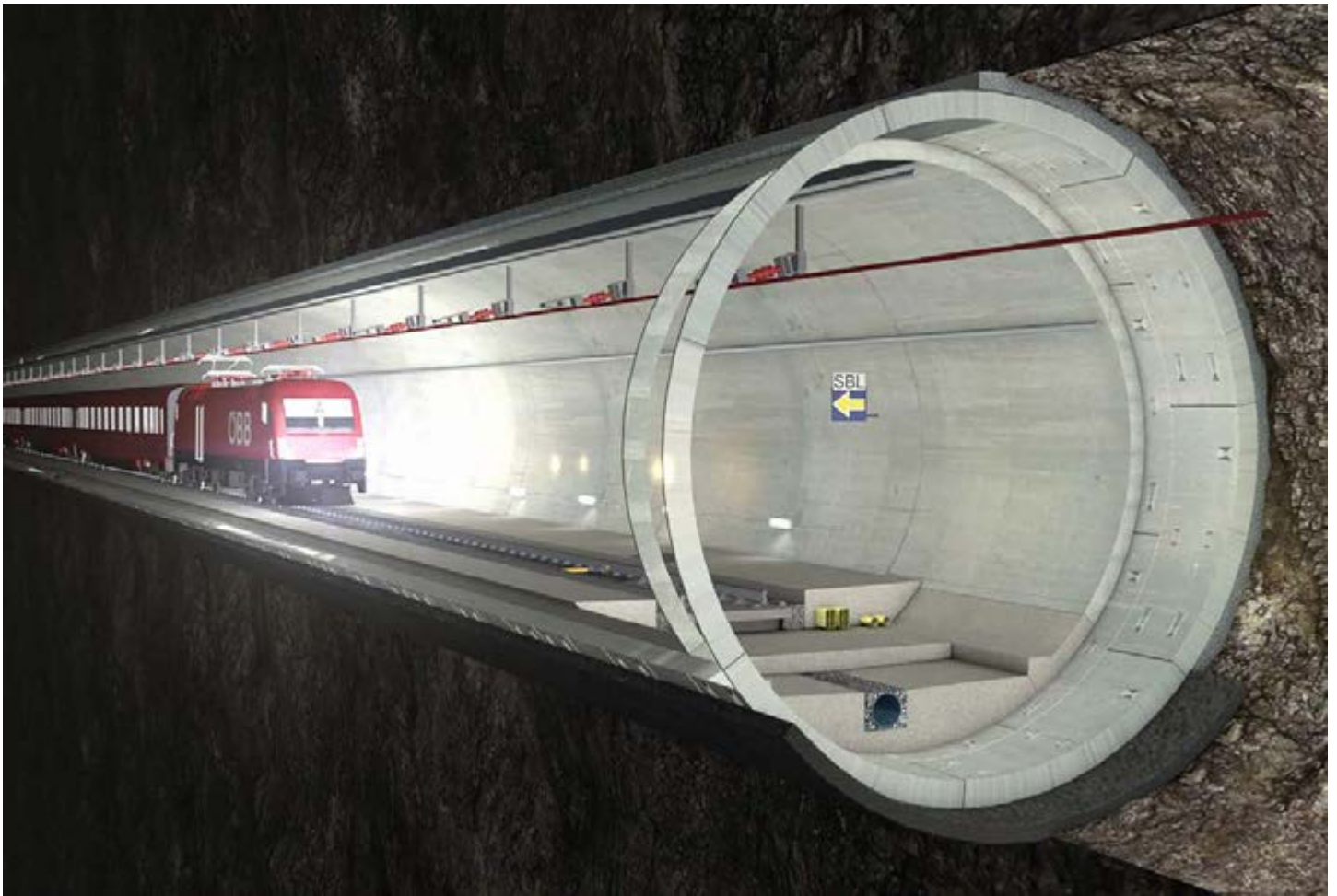
KORALMBAHN (Koralmbahn Railway). Through modern tunnels in about 45 minutes from Graz to Klagenfurt – environmentally friendly and faster than the car
