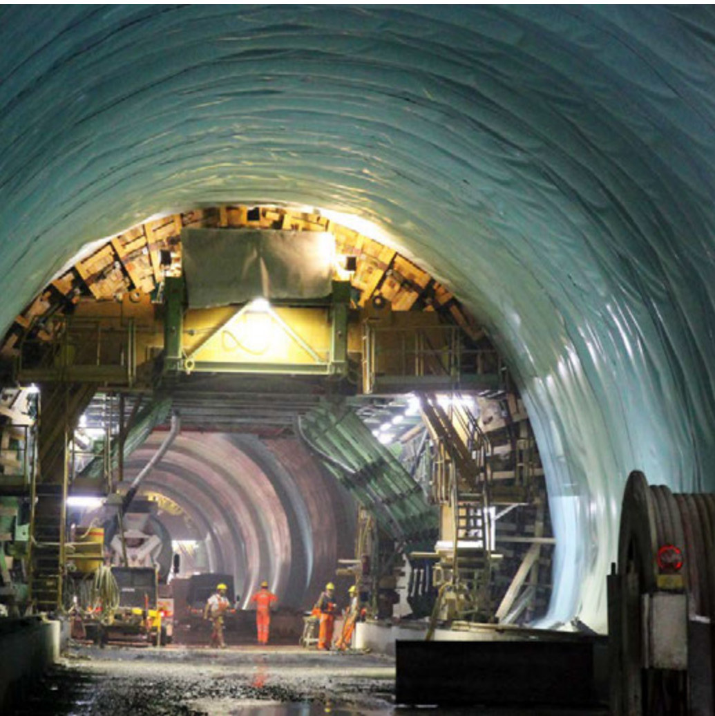
flows, ice forms. This means that tunnels need constant monitoring.
