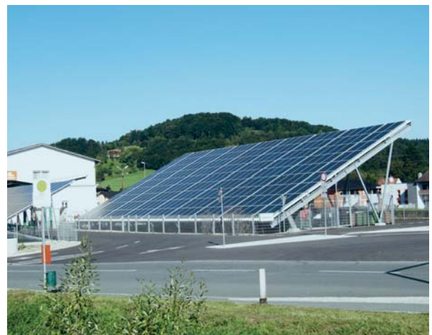
FELDBACH TRAIN STATION. First carbon-neutral train station in Austria, with 600 m 2 photovoltaic system
