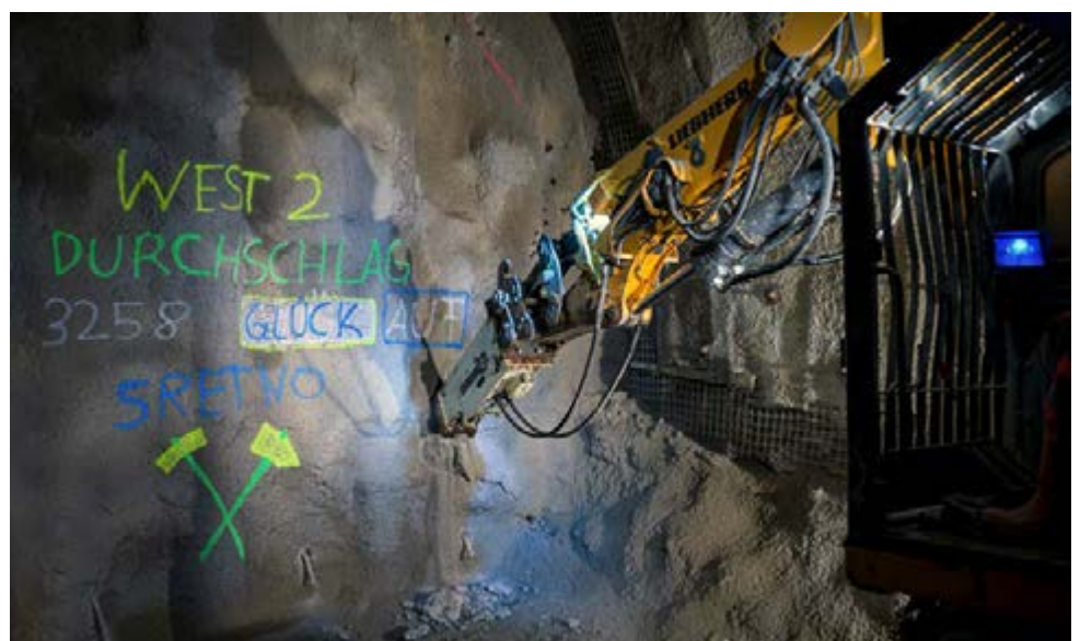
THROUGH THE MOUNTAIN. The last breakthrough in the Semmering Base Tunnel
