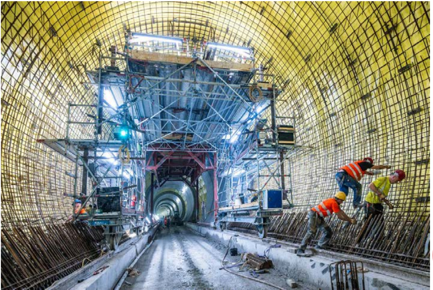
SEMMERING BASE TUNNEL While the final metres are still being excavated, the interior work is already progressing rapidly
