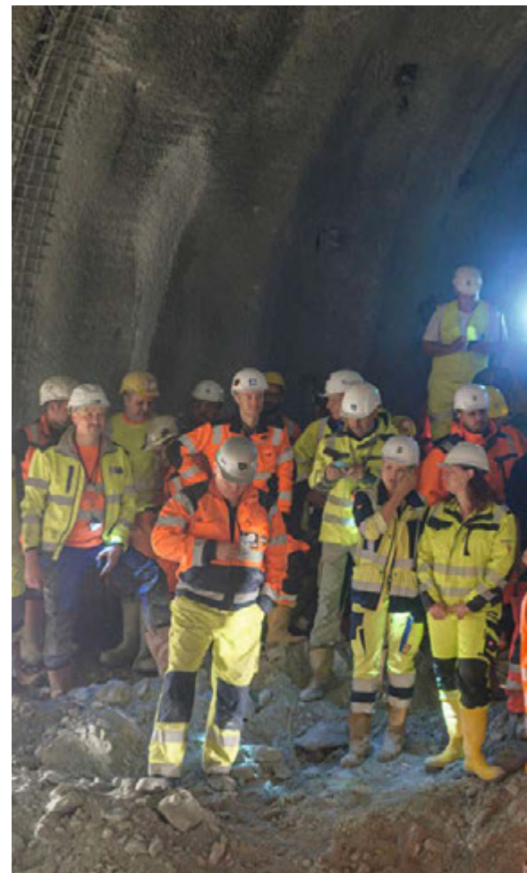
SEMMERING BASE TUNNEL In June 2022, the first
